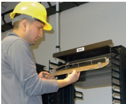
Side-in trays tilt outward to improve accessibility
