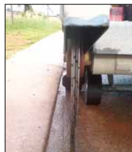
Slot Cutting / Microtrenching
